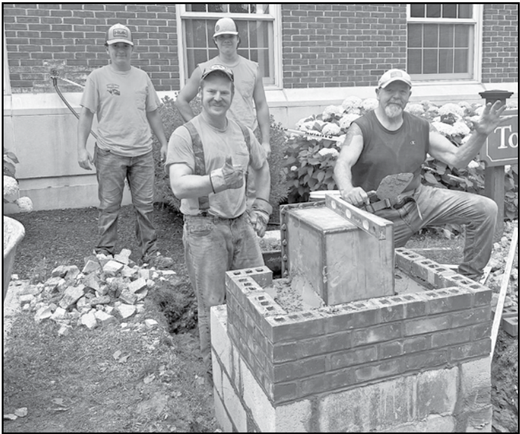
Kent Highway Department members who helped build the base for the statue include Jack Diskin, Tyler McMath, James Nix, and Highway Superintendent Richard Othmer.
