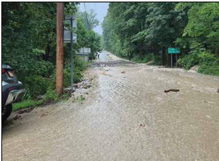
Flooding closed this road in Philipstown. Photos courtesy of CSFC.
